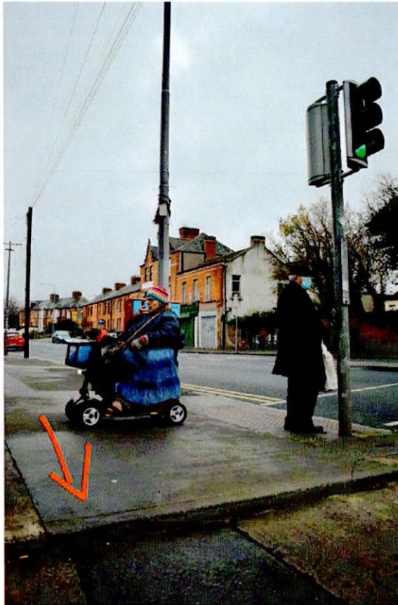
Steps at access to side roads force mobility aid users to use the road as they cannot proceed on the footpath (location at junction with Kilmainham Bank)
